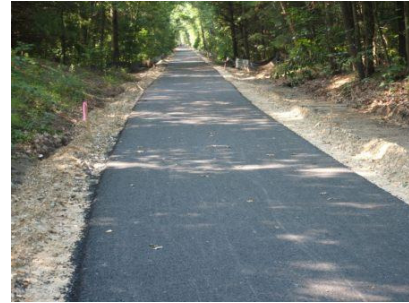
Newly constructed portion of the Derry Rail Trail. www.derryrailtrail.org
